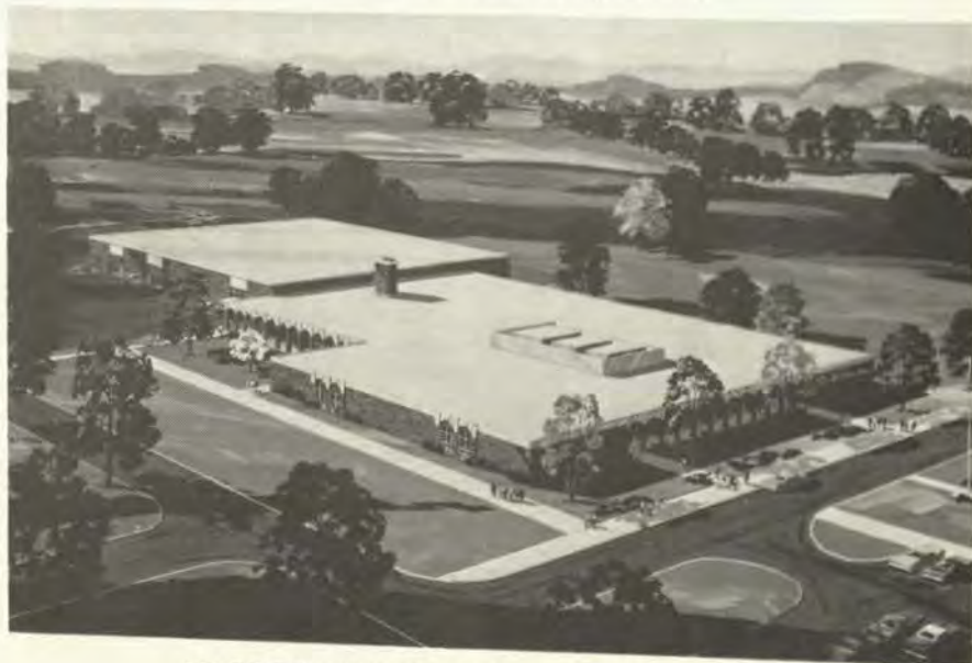
KNOX COUNTY JOINT VOCATIONAL SCHOOL
