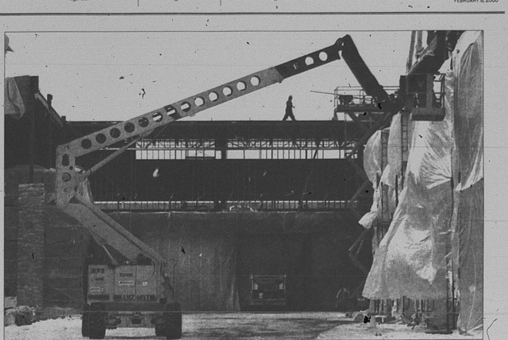
Construction is continuing on the 240,000-square-foot Cabela's store expected to open this fall at M-50 and US-23 near Dundee. The coming of the huge retailer has spurred the formation of a small business association in the village.
